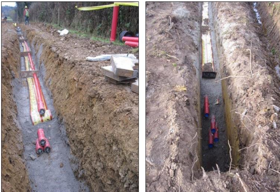
Plate 4-7 Typical Cable Trench View
