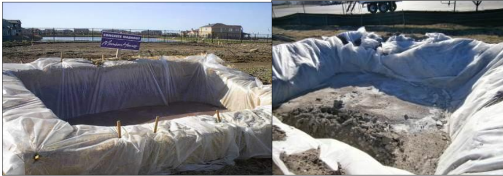
Plate 4-3 Concrete washout area
