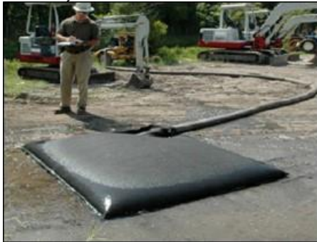
Plate 4-5 Silt Bag with water being pumped through
