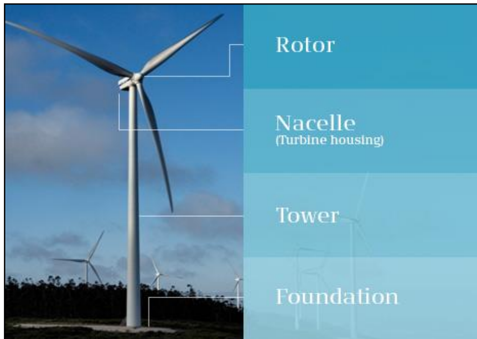
Plate 4-1 Wind turbine components
