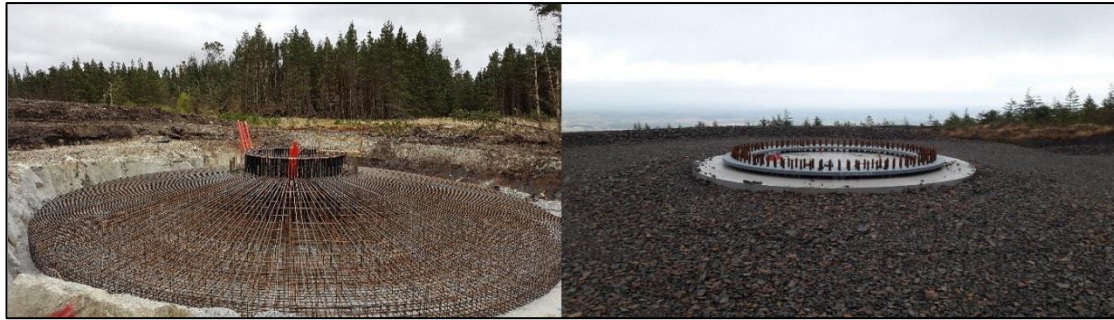
Plate 4-2 Turbine 'Anchor Cage' and finished turbine base
