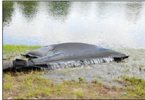
Plate 4-6 Silt bag under inspection
